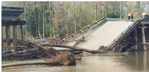
Figure 2: Bridge collapse due to debris buildup and pier foundation scour (HEC-09).
