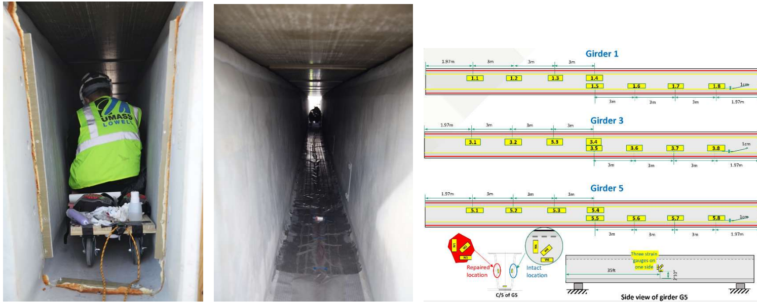
Figure 8. (a) Sensing textile installation scheme and (b) result (c) Design of integrated sensing textiles.
