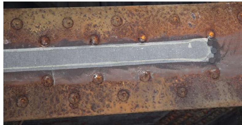
(a) Example extension end of sensing textile (from SFR Bridge, NH). (b) Example round end of sensing textile (from SFR Bridge, NH).
