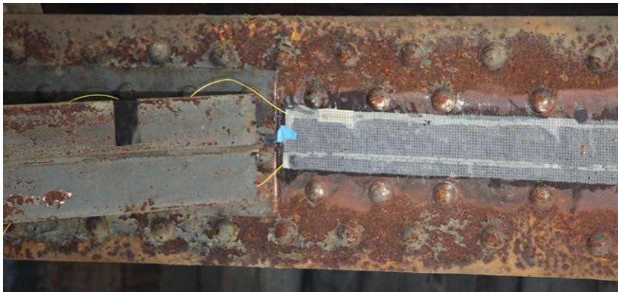
(a) Example extension end of sensing textile (from SFR Bridge, NH). (b) Example round end of sensing textile (from SFR Bridge, NH).
