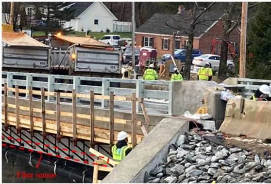
a) Installed optical fiber sensors b) Layout of optical fiber sensors
