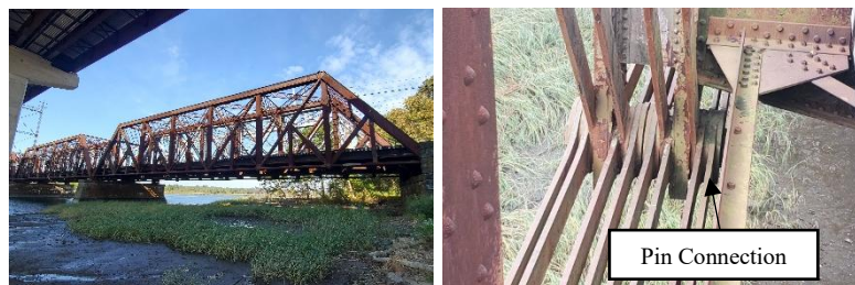
Figure 1 -Devon Bridge Span 7 (left), and Eye-bars Pin Connection (right)
