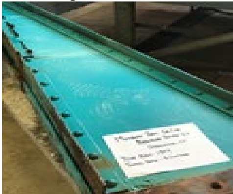
Figure 1: Brackets from Cos Cob Bridge in Greenwich, CT
