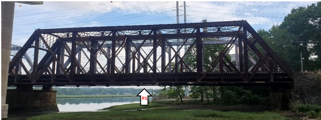
Figure 1 – Devon Bridge (CT), Span 7, P1 location
