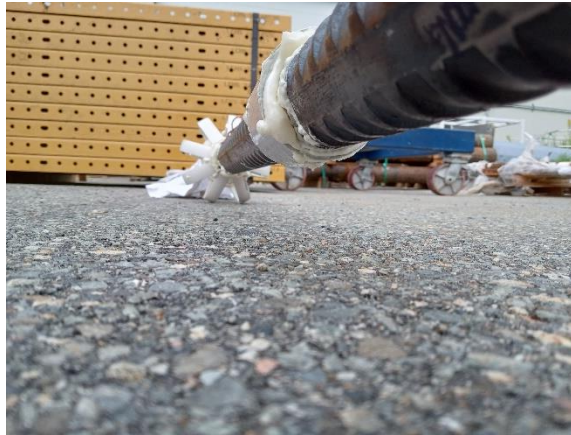
Figure 2 Specimen assembly process: Instrumented reinforcing bar at the job site.
