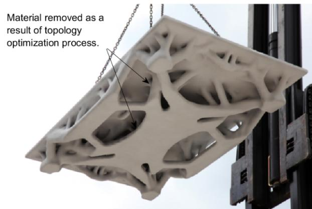
Figure 2: Topologically optimized slab cast using 3D printed formwork being placed [2]
