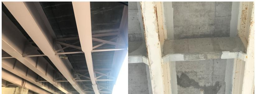
Figure 1: Cross frames on the left and concrete diaphragm on the right.
