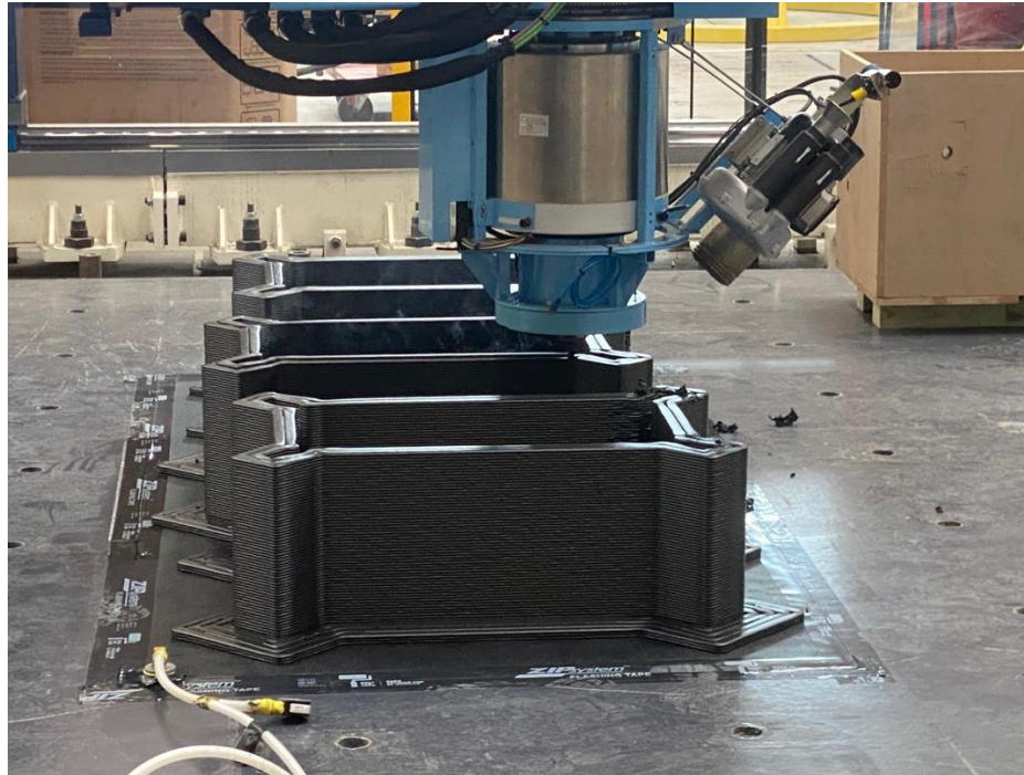
Figure 1 – CF-ABS formwork being printed using Ingersoll MasterPrint.
