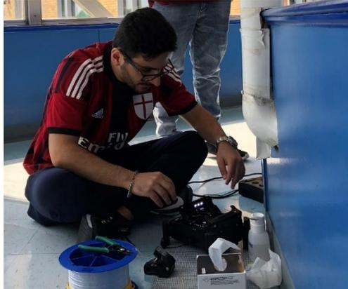
Figure 5. Extending sensing fiber cable to an optical fiber spool and connection fiber cable.
