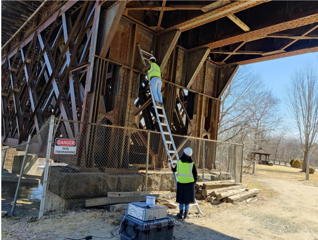
Figure 1 Field test under the Salmon Fall River Bridge in March 2022.
