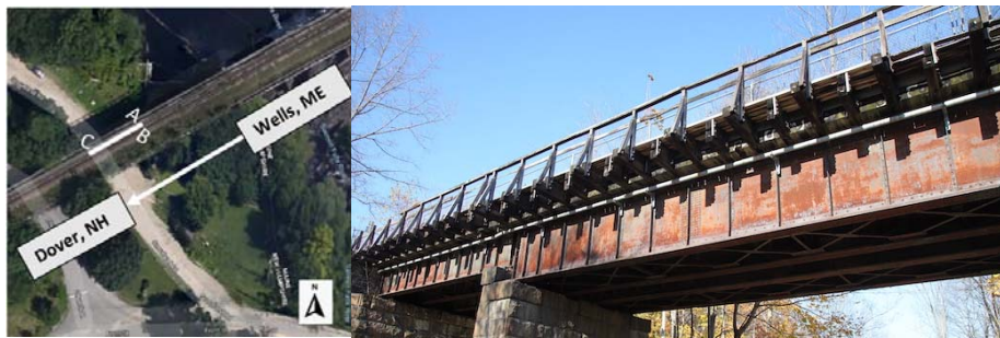
Figure 1. Salmon Falls River bridge in South Berwick
