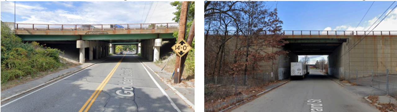
a) I-495 bridge in Chelmsford
