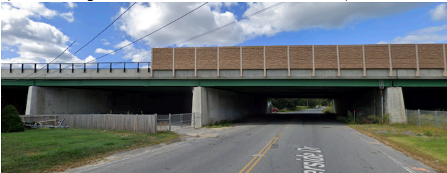
c) I-93 bridge in Methuen
