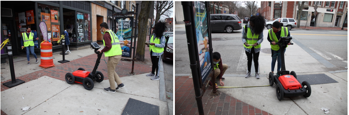
Fig. 2 a) GPR inspection of concrete slabs
