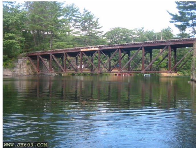
Figure 2. – Tilton Belmont RR Bridge, NH
