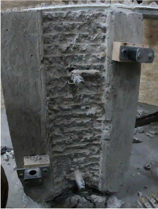
Figure 30: Specimen 4 – Concrete Ridge Shear Failure and Spalling
