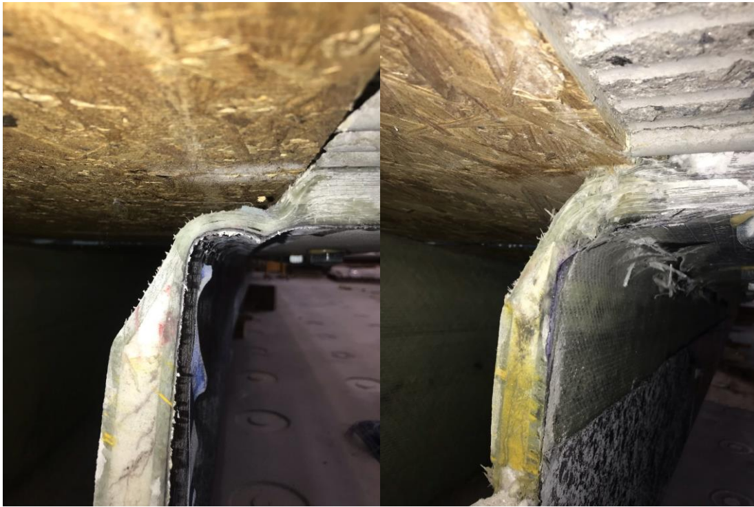
Figure 72: Top Flange Radius Buckling (Left) and Delamination (Right)
