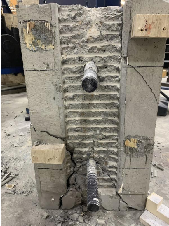
Figure 21: Specimen 1 – Concrete Crushing Failure
