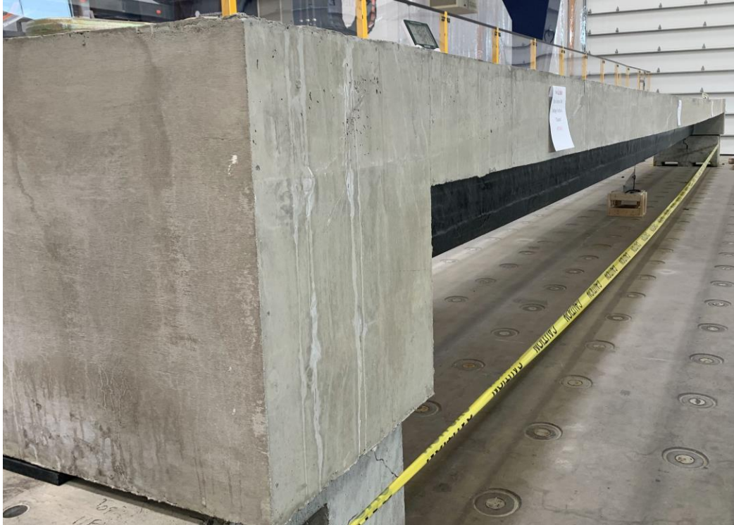
Figure 38: UTC-1 Creep Girder Specimen
