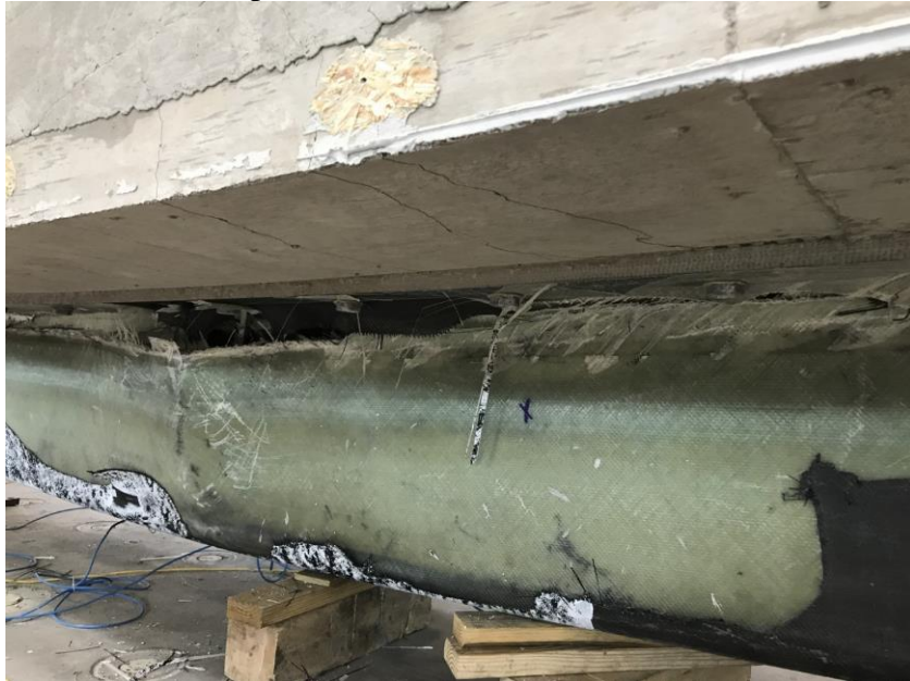
Figure 71: UTC-2 After the 253 kip Failure Load
