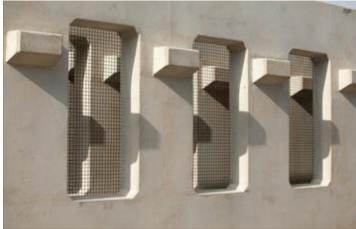
Figure 1. Window openings in precast concrete wall panels with Litewall pedestrian screening (patented by Unistress).
