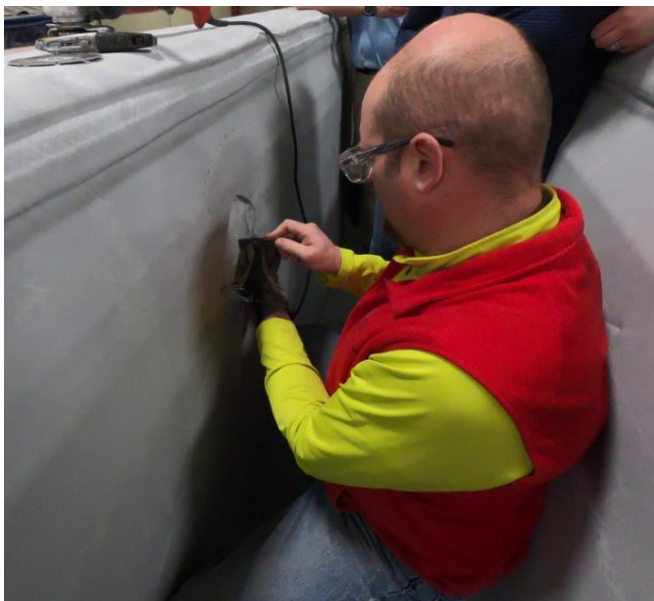
Investigation of Girder Defect
