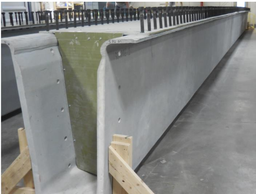
Fully infused, cured, and post-processed FRP tub-girder
