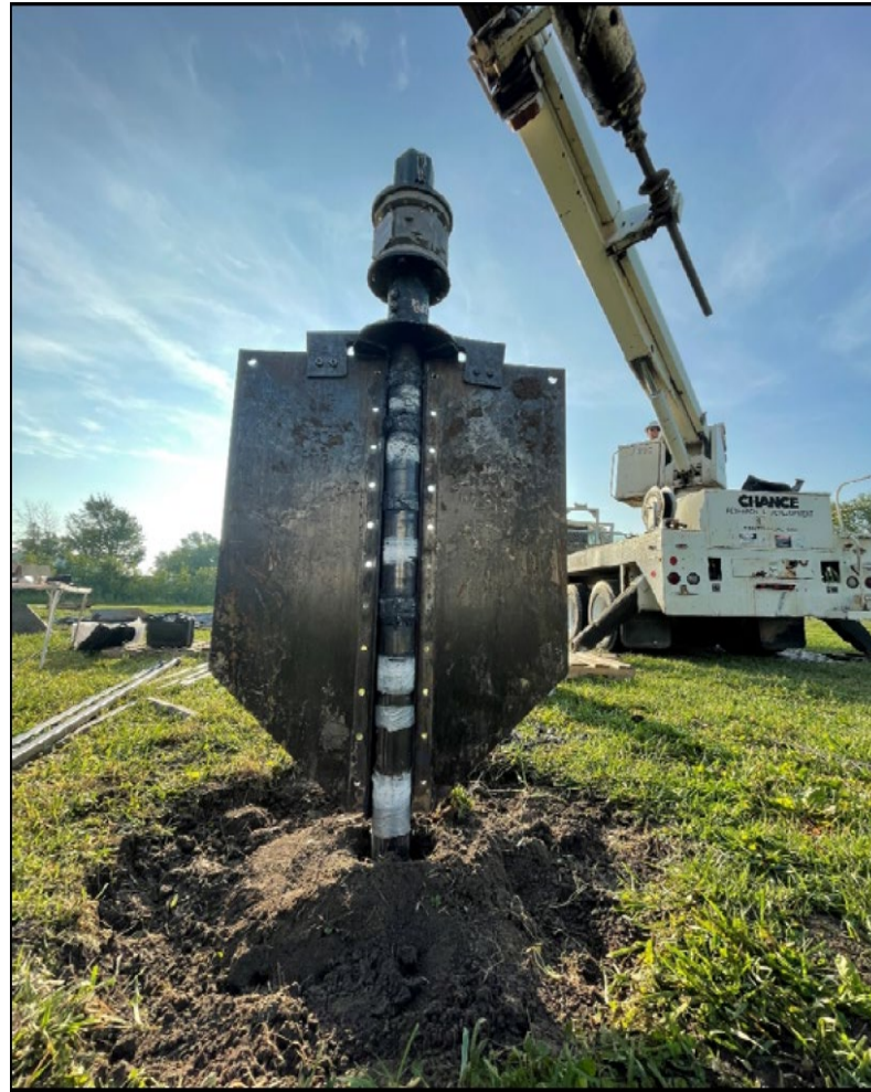
Figure 6. CV 36-36 before installation in the ground. (Vane diameter= 0.9, Total Height = 1.2 m)
