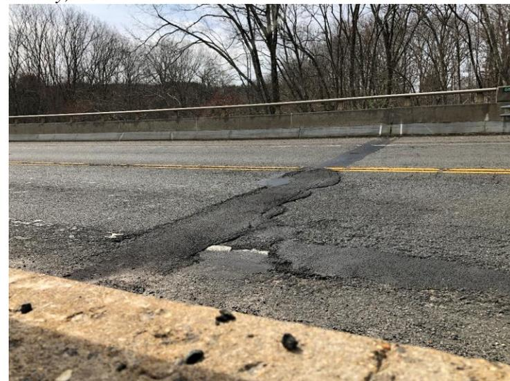
Figure 2. Expansion Joints (a) side view, (b) through view, (c) road way view (showing this is an asphaltic joint)
