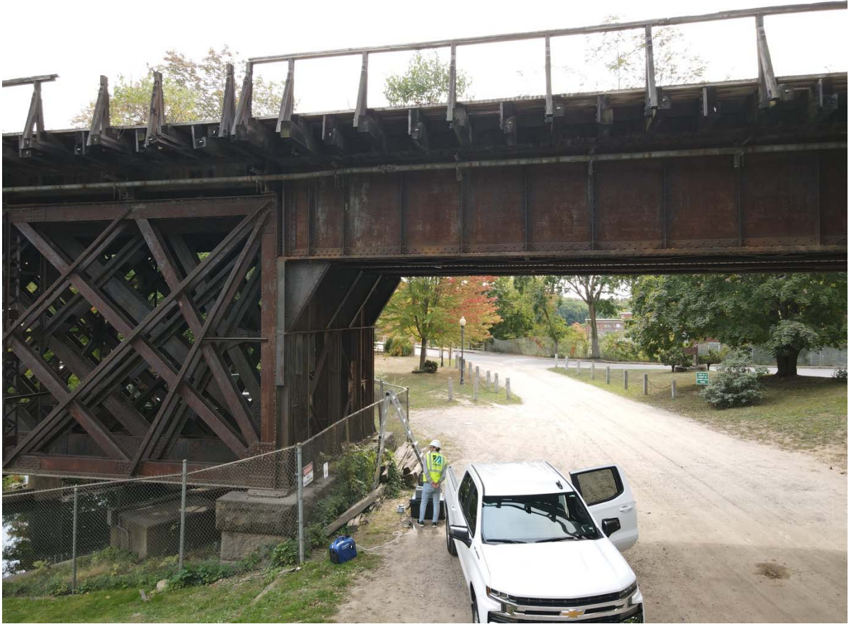
Figure 2 Photo of UML students collecting data under the bridge.
