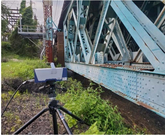
Figure 1 – Cos Cob Bridge: Horizontal reading vibrometer setup
