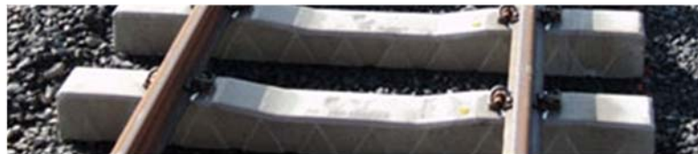
(a) Prestressed concrete crosstie
