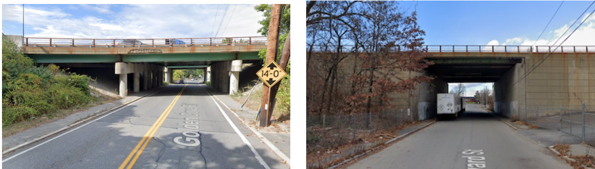
a) C-08-026 I-495 Bridge (Chelmsford) b) L-15-076 Rt. 3 Bridge (Lowell)
