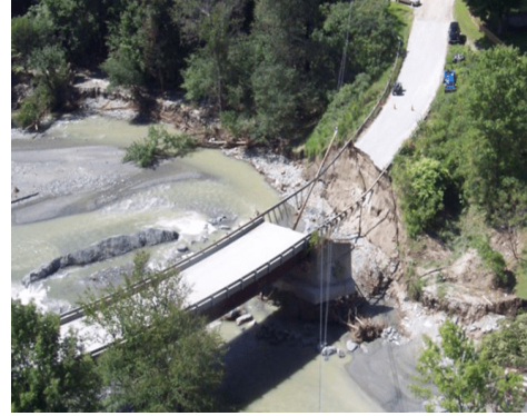
Vermont, USA - 2011 Tropical Storm Irene (Photo credit: VTrans; National Wildlife Federation, 2016)
