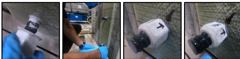
Figure 2-20: Applying Epoxy to the Shear Blocks
