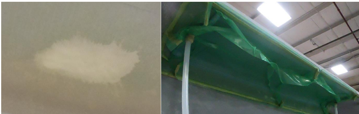
Figure 16: Right: Minor "Dry Spot" Surface Imperfection Left: Secondary Repair Infusion
