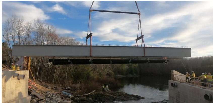
Figure 13: Two-Girder Unit Being Lifted into Place
