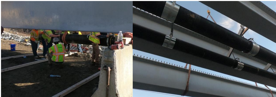
Figure 12: Utility Hangers (Left: Installation; Right: In Place)
