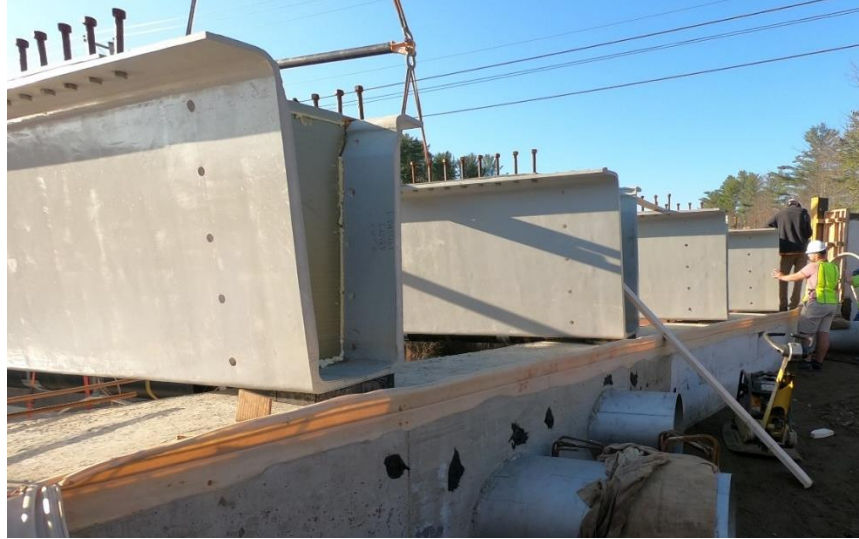
Figure 14: Girder Ends Placed on Bearing Pads
