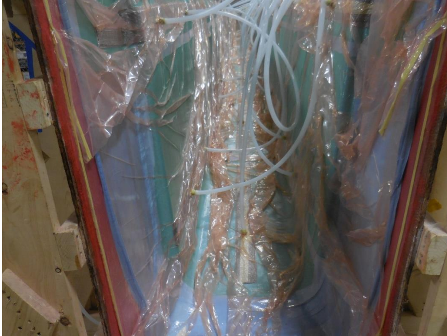
Figure 8: Consolidated Girder with Flow Media and Vacuum/Resin Feed Lines Visible
