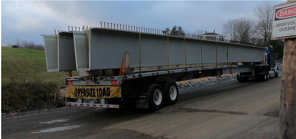
Figure 11: Girders Arriving at Bridge Site
