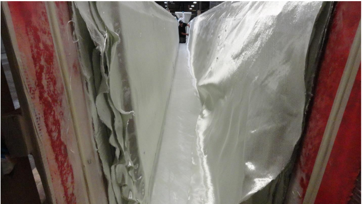
Figure 7: Layup of Girder Reinforcement in Process
