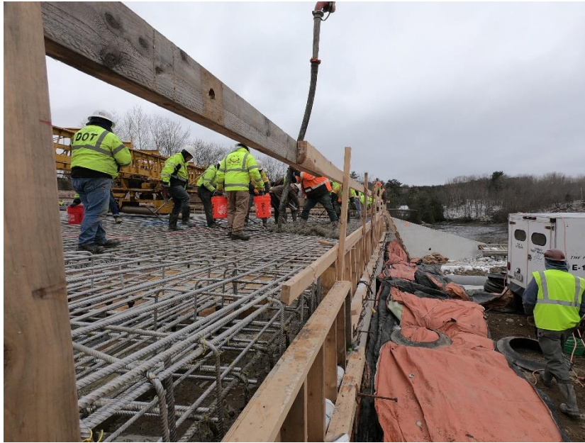
Figure 15: Reinforced Concrete Deck Pour
