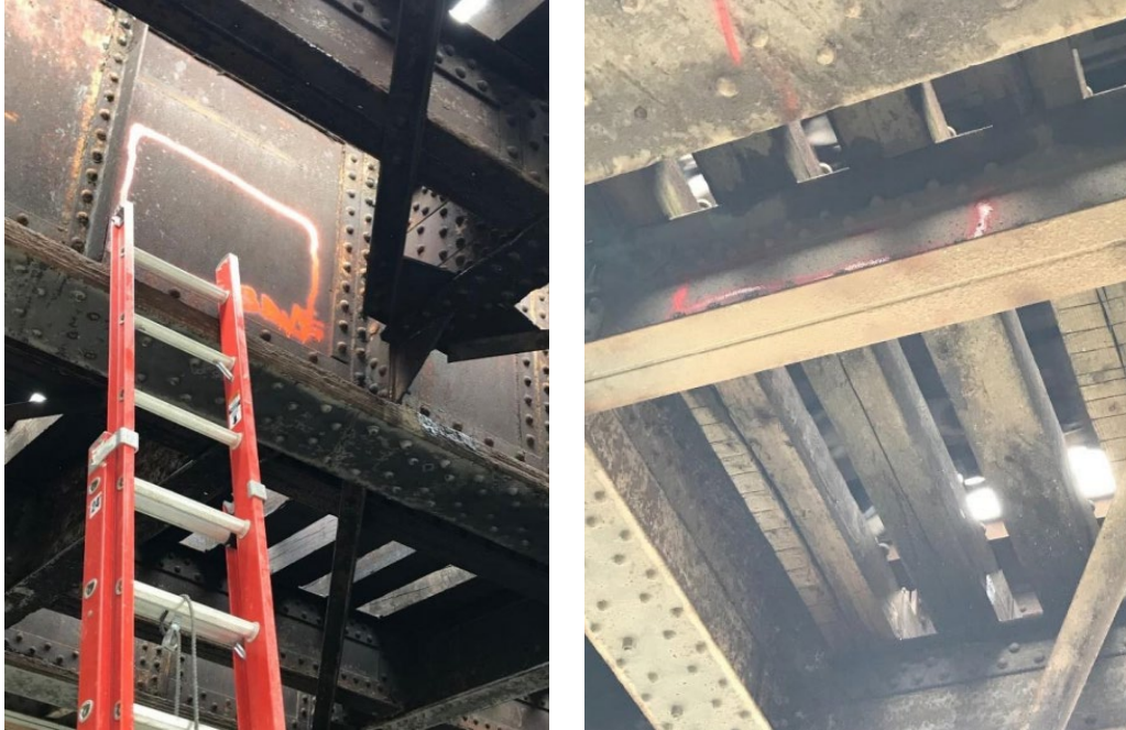
Figure 9: Girder material (left) and stringer material obtained from Atlantic Street Bridge, CT.
