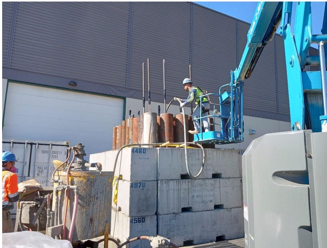
Figure 1 Specimen assembly process: Grouting of the steel casings in collaboration with Maine Drilling and Blasting (MD&B).
