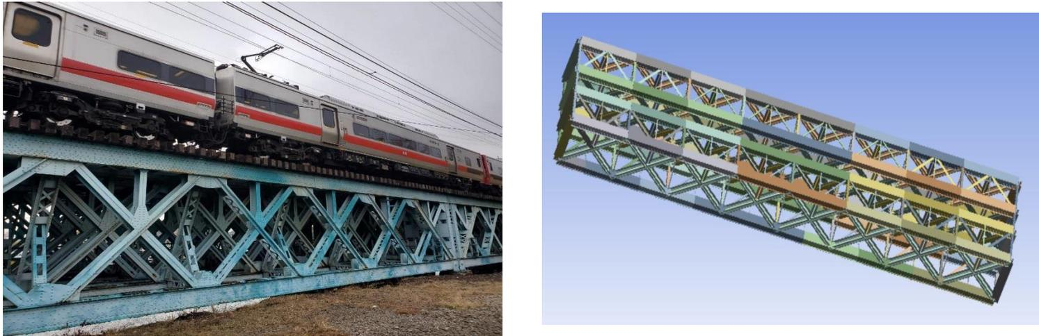
Fig. 1: Cos Cob Bridge, CT (Left) and preliminary FEM model of the bridge (right)
