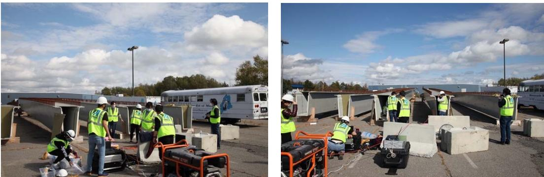
**Fig. 1.** Installation of sensing textiles on three composite bridge girders (10/06/2020)
