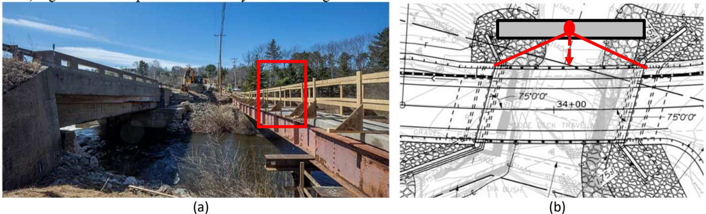
Figure 6. (a) Hampden Bridge in Maine and the planned location for data acquisition, (b) sketch of the temporary pedestrian bridge to set up video camera.
