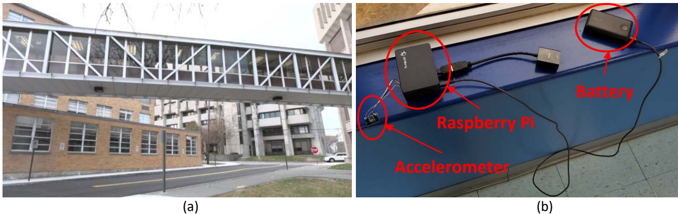
Figure 1. (a) Olney Hall bridge at UMass Lowell; (b) RaspberryPi data acquisition system.
