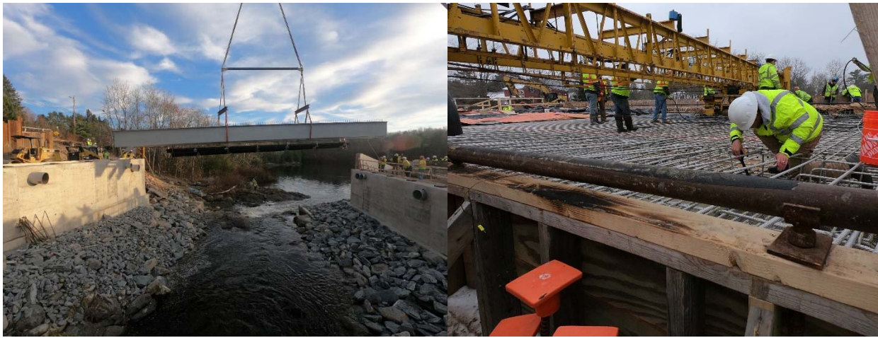
Left: First Girder Being Placed; Right: Preparation for Deck Pour
