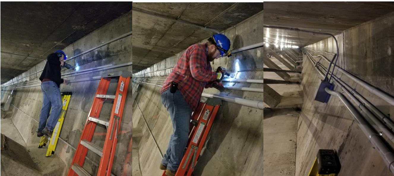
Figure 1 Fiber optic sensor conduit installation on the first span (A anchors) from the Prospect side of the PNB
