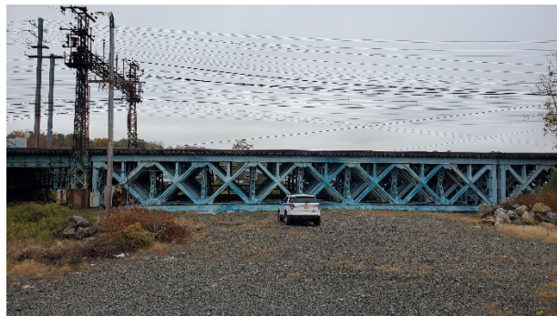
Figure 3 – Cos Cob bridge: Span 7 for Future Field Test
